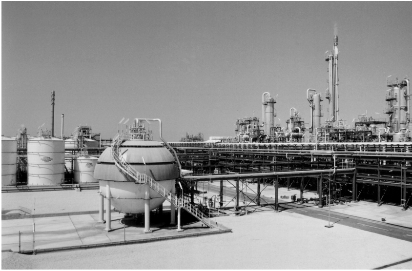
Figure 1.5 Chemical complex erected in Katar by UHDE GmbH, Dortmund, Germany. The chemical complex consists of three main plants for the production of 260 000 t/a chlorine, 290 000 t/a caustic soda, 175 000 t/a ethylene dichloride and 230 000 t/a vinyl chloride. The order value was approx. 450 million US$.
